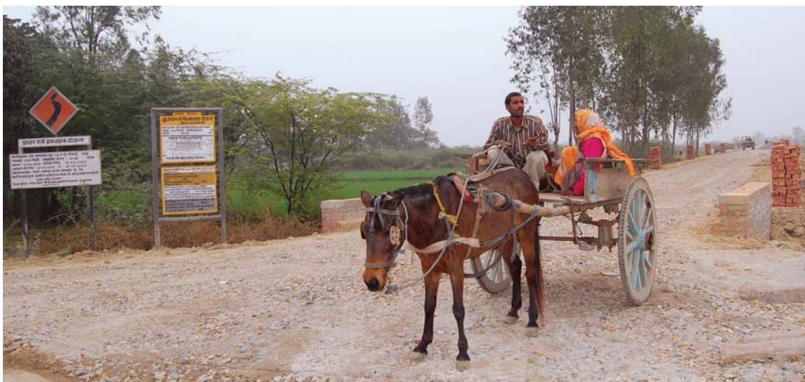
Already in use - a road being constructed under PMGSY
