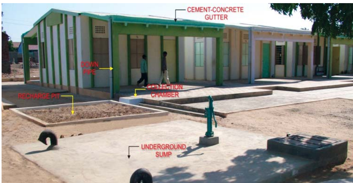
Rainwater Harvesting in Institutions
