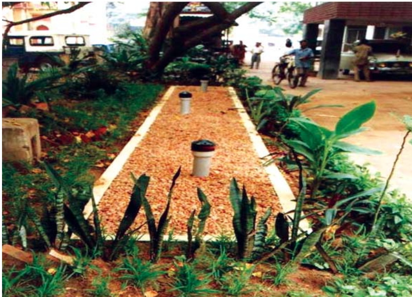
Sustainability measures - Recharge Shafts for Ground Water
